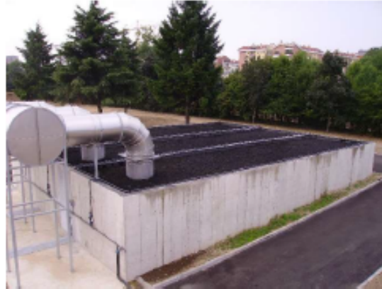
Figure 1 - Mónafil Installation in Milan, Italy
